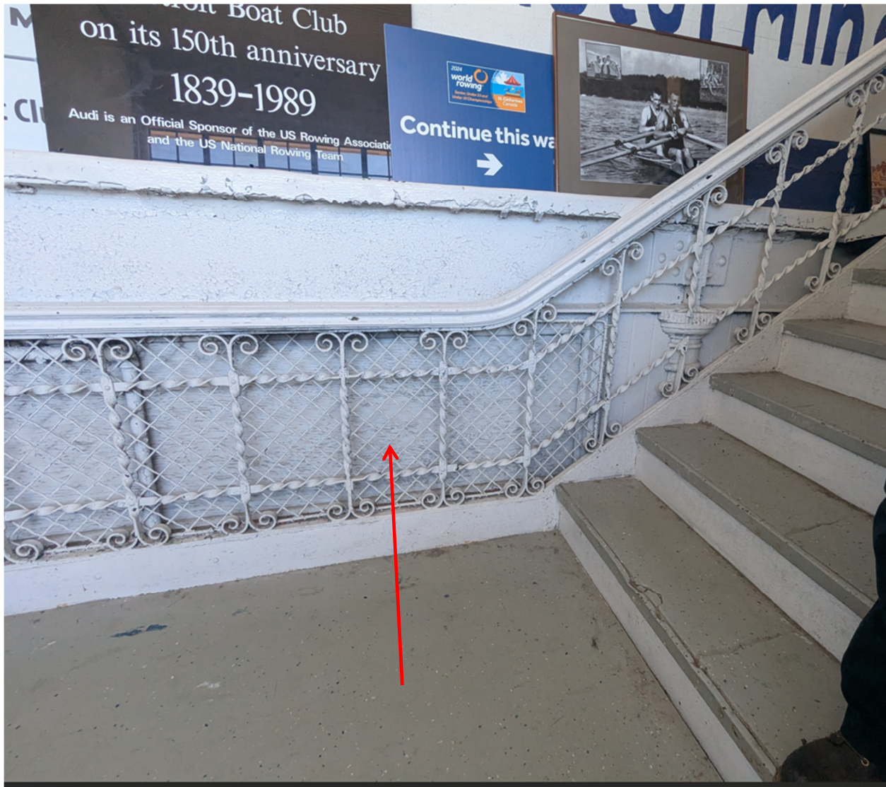
Photo 2: Wood Panel to be replaced with pre-finished insulated metal panel.
